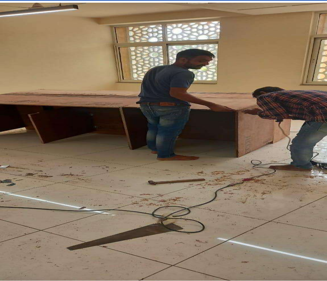
Academic Block-2 room no-27 furniture work
