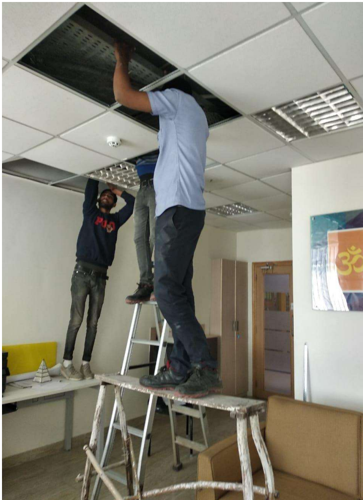
AC Unit installation in Purchase Office
